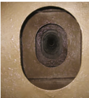
Second coat - PERMA FILM Buff with 250 µm (wff.)
